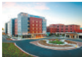
PHOTO COURTESY OF HARBISON-MAHONY-HIGGINS BUILDERS INC. Kaiser Permanente South Sacramento Medical Center was constructed by HMM Builders Inc.
