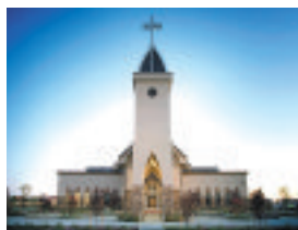
PHOTO COURTESY OF HILBERS INC. The 14,670-square-foot St. John's Episcopal Church — Roseville was built by Hilbers Inc. and cost $3.6 million.
